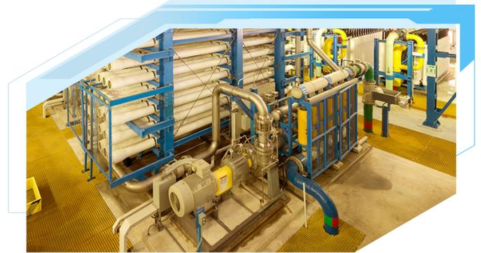
These systems require a range of parts such as bearings that can withstand corrosion caused by high pressure flow of seawater and sand. The materials used for these parts can greatly influence component lifespan and operational costs. Components made with alumina ceramic provide superior performance over those made from metals.
